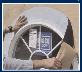
Protecto Flex® is a 40-mil thick peel and stick flashing tape. The flexible cross-laminated top surface will expand and conform to irregular or curved surfaces while the aggressive adhesive forms a permanent bond between the window fin and the building substrate. Protecto Flex gives you a total air and water seal without having to cut and patch in the membrane to conform to irregular or curved window and door openings.
